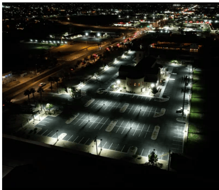
Figure 1: above represents the outcome of retrofitting with COB LED's. You will notice very uneven lighting with hot spots and dark spaces in the parking area.
